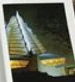
Shard's glass facade The glass facade of the Shard is made of 10,000 glass panels, each of which is 1.5m x 1.5m.
